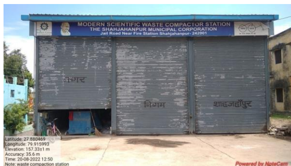
Figure 35: Waste segregation unit at Jail Road near fire station
