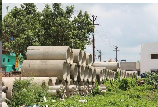
Figure 31: STP construction and laying of underground sewer line in progress
